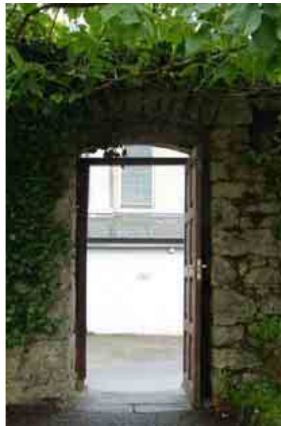
Gateway Through Wall
