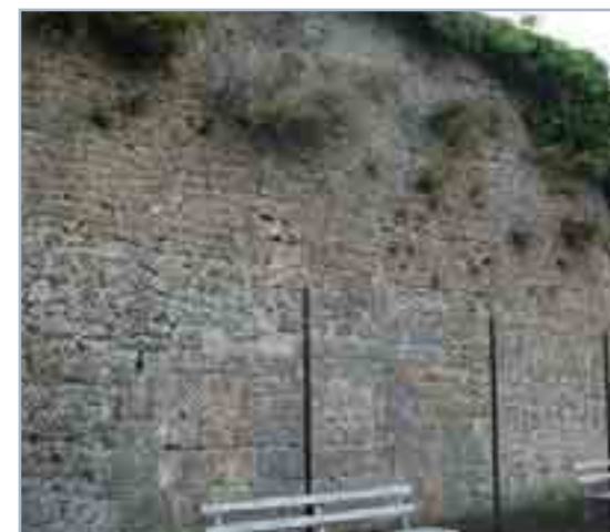
Wall at GAA pitch
