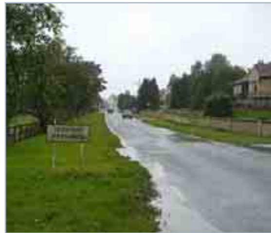
Lack of Pavements
