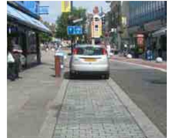
On-street Parking Bays/ Bollards
