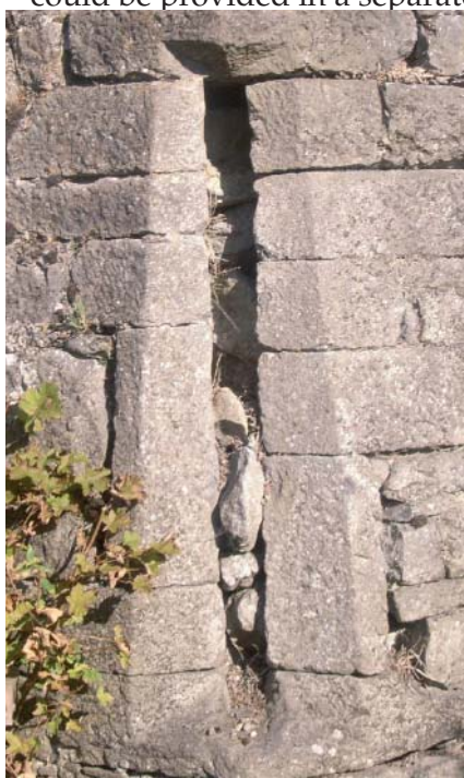
Figure 13: Watergate arrow slit
